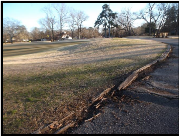
Photo 9: Wood edgers are damaged and deteriorated.
