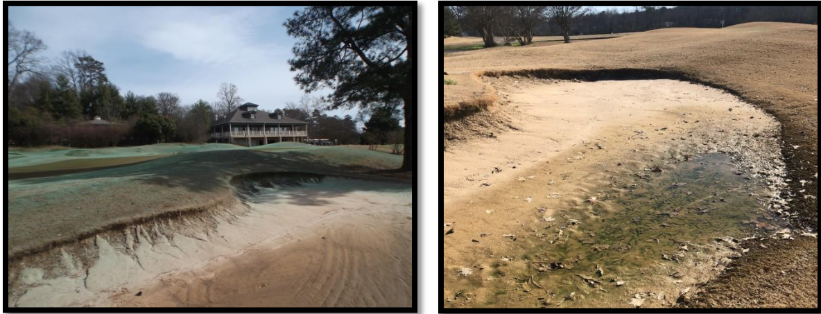
Photo 7-8: Bunkers have eroded edges, contaminated sand, and poor drainage.
