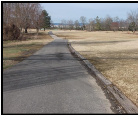
Photo 11-12: Deteriorated railroad tie cart path edging and retaining walls are unsightly.
