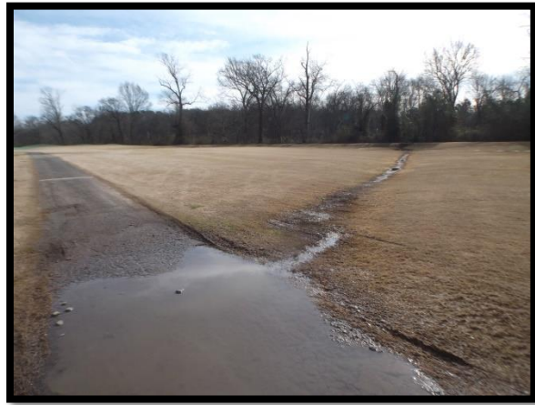
Photo 5: Flat fairways and pockets of standing water. Photo 6: Shallow grass swales drain poorly.
