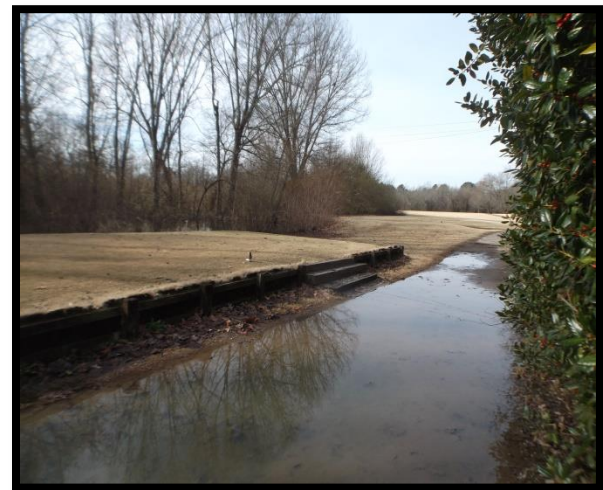
Photo 11-12: Deteriorated railroad tie cart path edging and retaining walls are unsightly.
