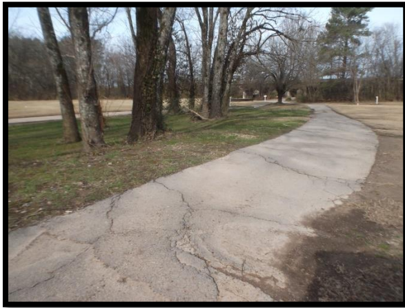
Photo 9-10: Deteriorated cart paths should be replaced.
