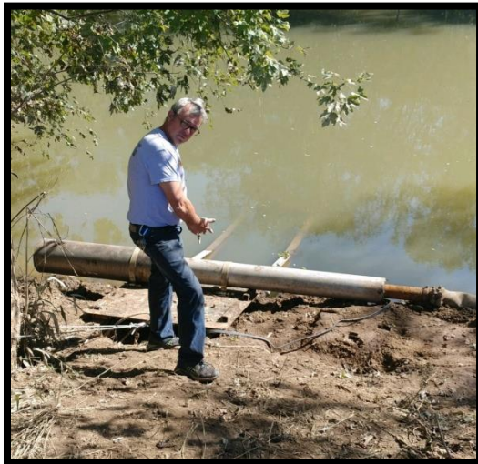
Photo 2: A single 40 horse vertical turbine pump lies on its side in the river. The second pump failed and was never replaced.
