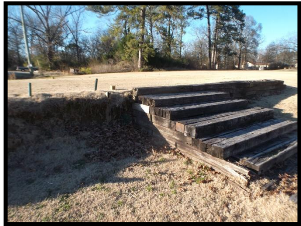
Photo 10: Railroad ties are rotten and falling down.
