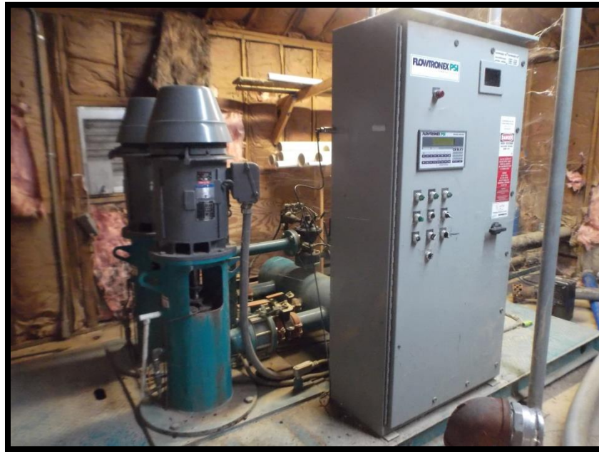
Photo 3: Modern vertical turbine pump station is adequately sized and is in good condition.
